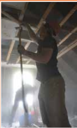
Two-family home under construction at 6-8 First Street
