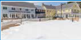
Assisted Living facility, 149 County Road
